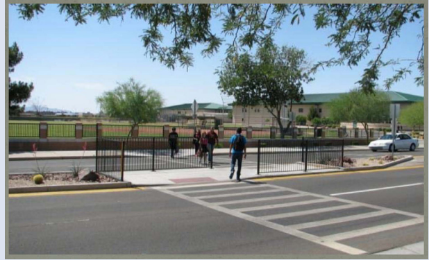
A midblock crosswalk was designed to accommodate students crossing an arterial to get to food establishments. Students were not using the pedestrian crossing 600 ft. away.
