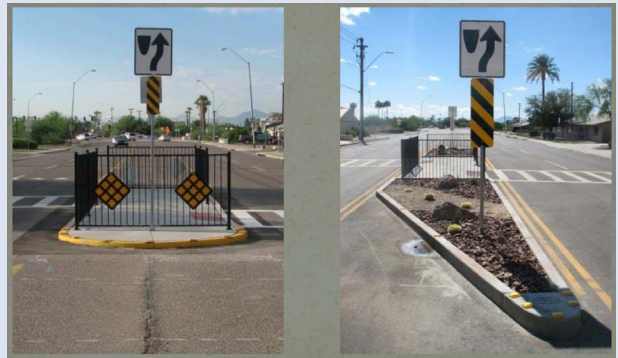
Before and after: Landscaping was added to crossing refuge.
