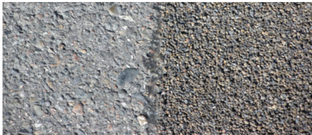
Untreated asphalt pavement is shown on the left. High friction surface treatment, with its sandpaper texture, is on the right.
