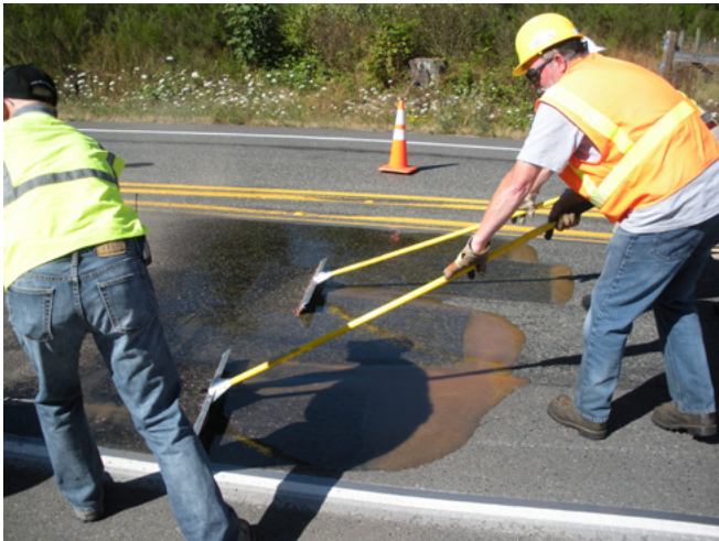
A Thurston County, WA, crew places calcined bauxite aggregate over an acrylic resin binder at this HFST project in 2014.
