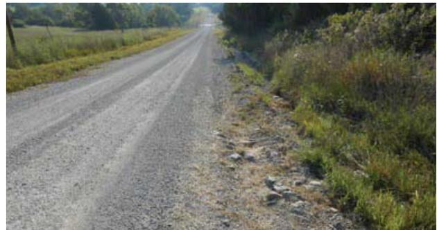
Fig 7. Inadequate ditch evidenced by washing along shoulder.
