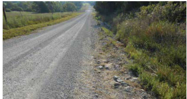
Fig 7. Inadequate ditch evidenced by washing along shoulder.
