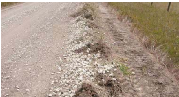
Fig 6. Improper mixing of dirt with windrow when repairing a high shoulder.
