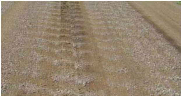
Fig 9. Washboards are common in dry weather.
