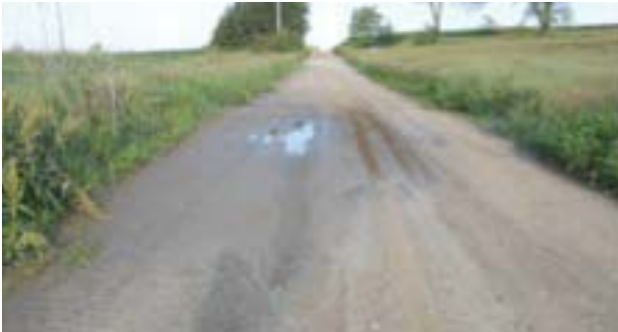
Fig 5. High shoulder causes mud hole at low spot.
