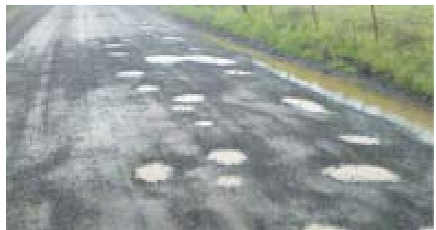
Fig 8. Potholes caused by inadequate cross slope at low spot in road.
