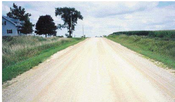
A well-maintained rock road has a four to six percent slope (crown) with a good crust and minimal loose material.
