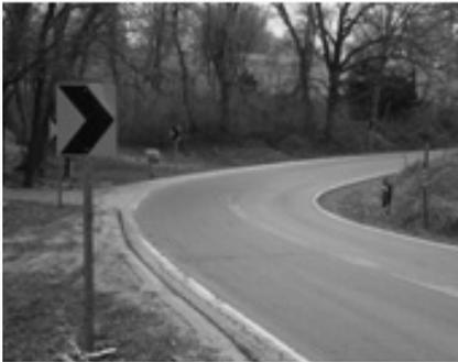
*A high friction surface treatment was added to the outside lane of this curve on K5 highway in 2009 in Leavenworth County.*
