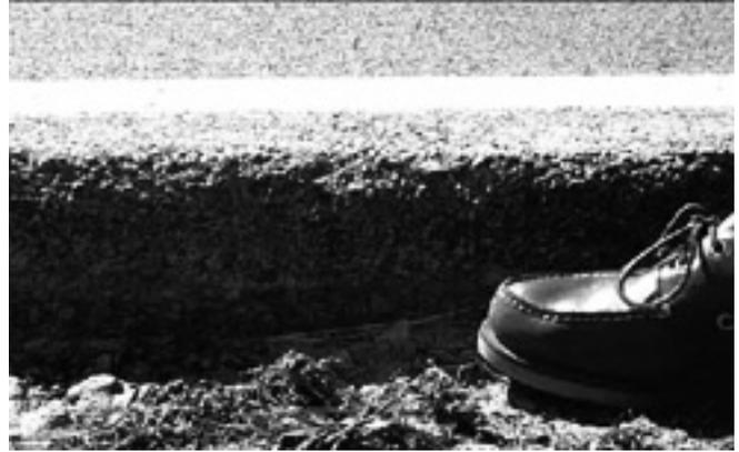
*A pavement edge without the Safety Edge has an abrupt drop-off that makes it more difficult for errant vehicles to recover back to their lane without over-correcting.*
