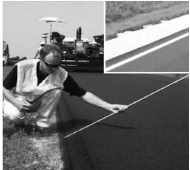
*This shows the Safety Edge during an overlay project and the finished product with the shoulder material in place next to the Edge (inset).*
