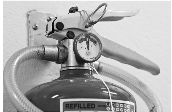
Two indicators of an extinguisher's charge are the pressure gauge and the plastic tie holding the pin in the handle.
