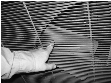
Photos courtesy of Riley County
