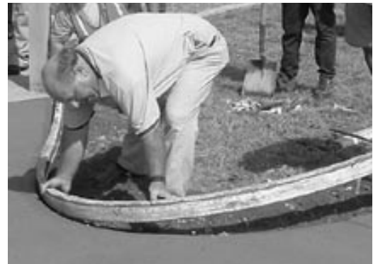
Forms are flexible and can be easily removed.
