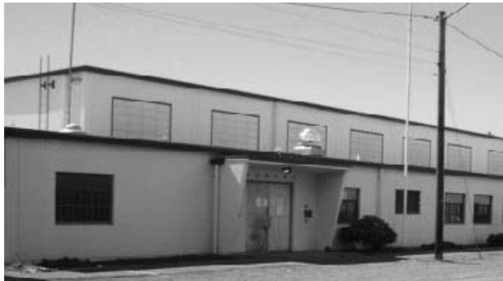
Mason Transit in Shelton, WA, purchased the downtown Shelton Armory with plans to develop a combined community center and expanded transit center.
