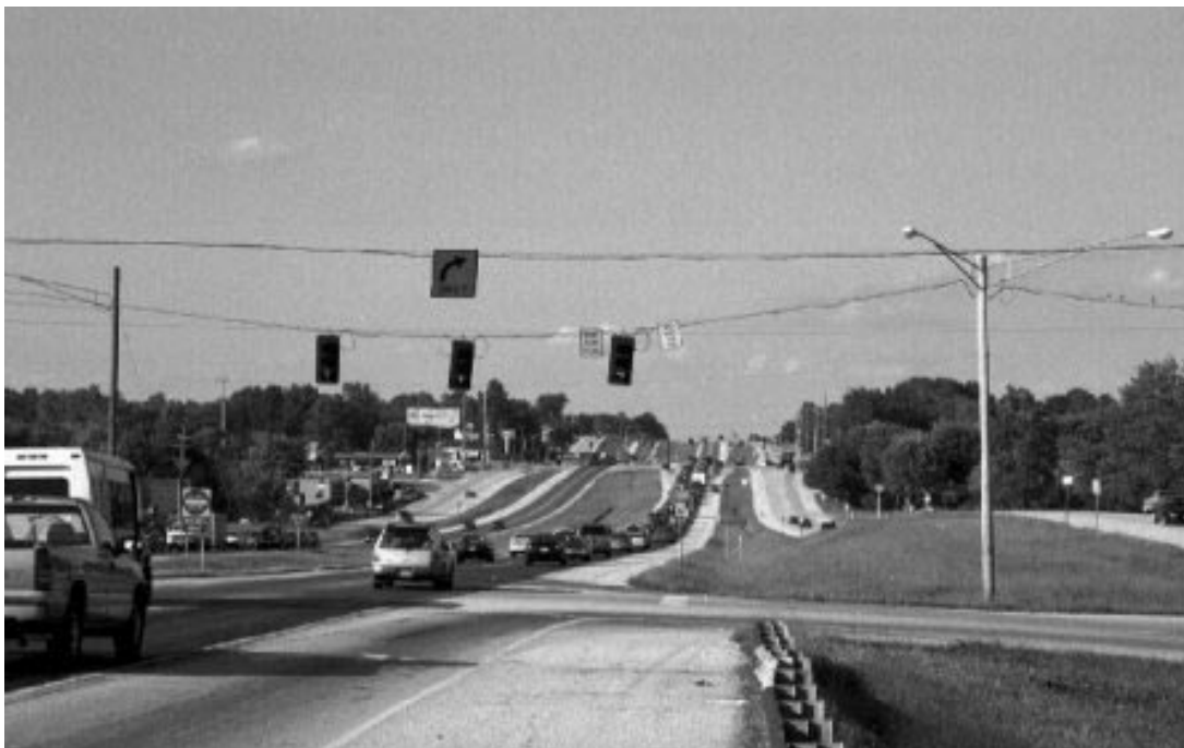
◀ Figure 6. View of Route 367
